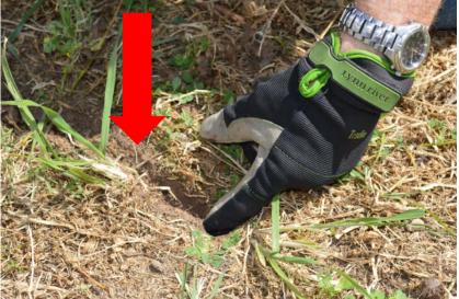
Use a small trowel to dig a trench to accept the probe cable. During excavation, place your finger over the hole to prevent any soil falling in.
