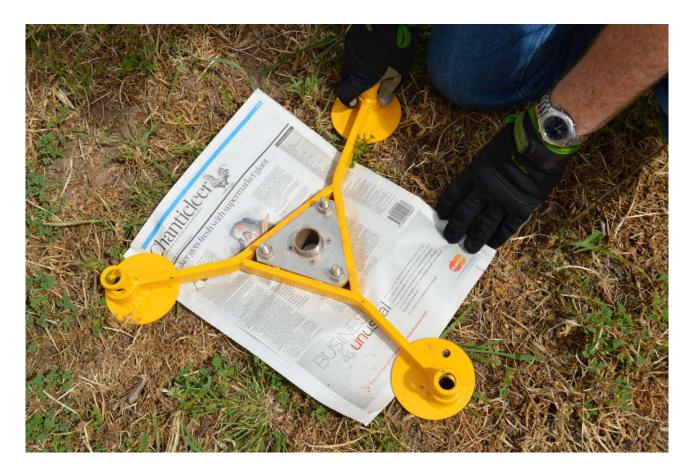
Place 2 sheets of newspaper beneath the Stabilisation Tripod. This allows easy removal of the augered soil later.
