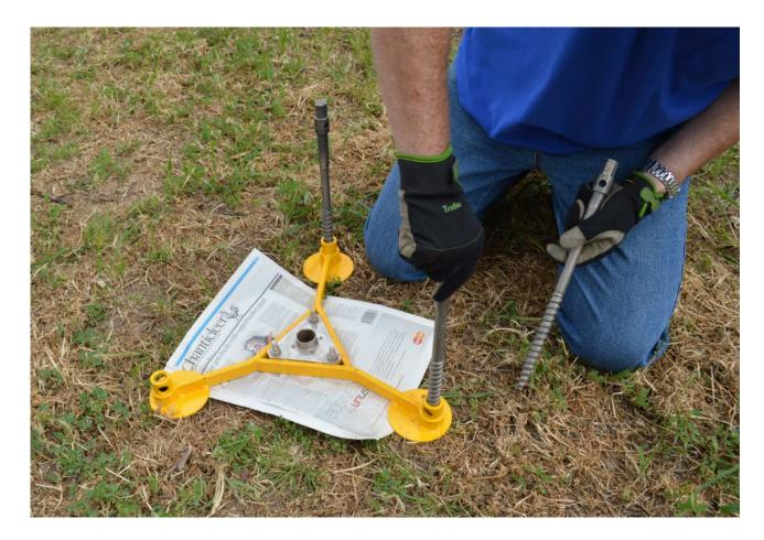
Insert the Screw Pins.
