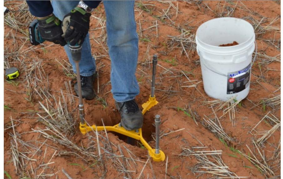
Position the Extension Tube in the centre of the excavated hole and install the Screw Pins.
