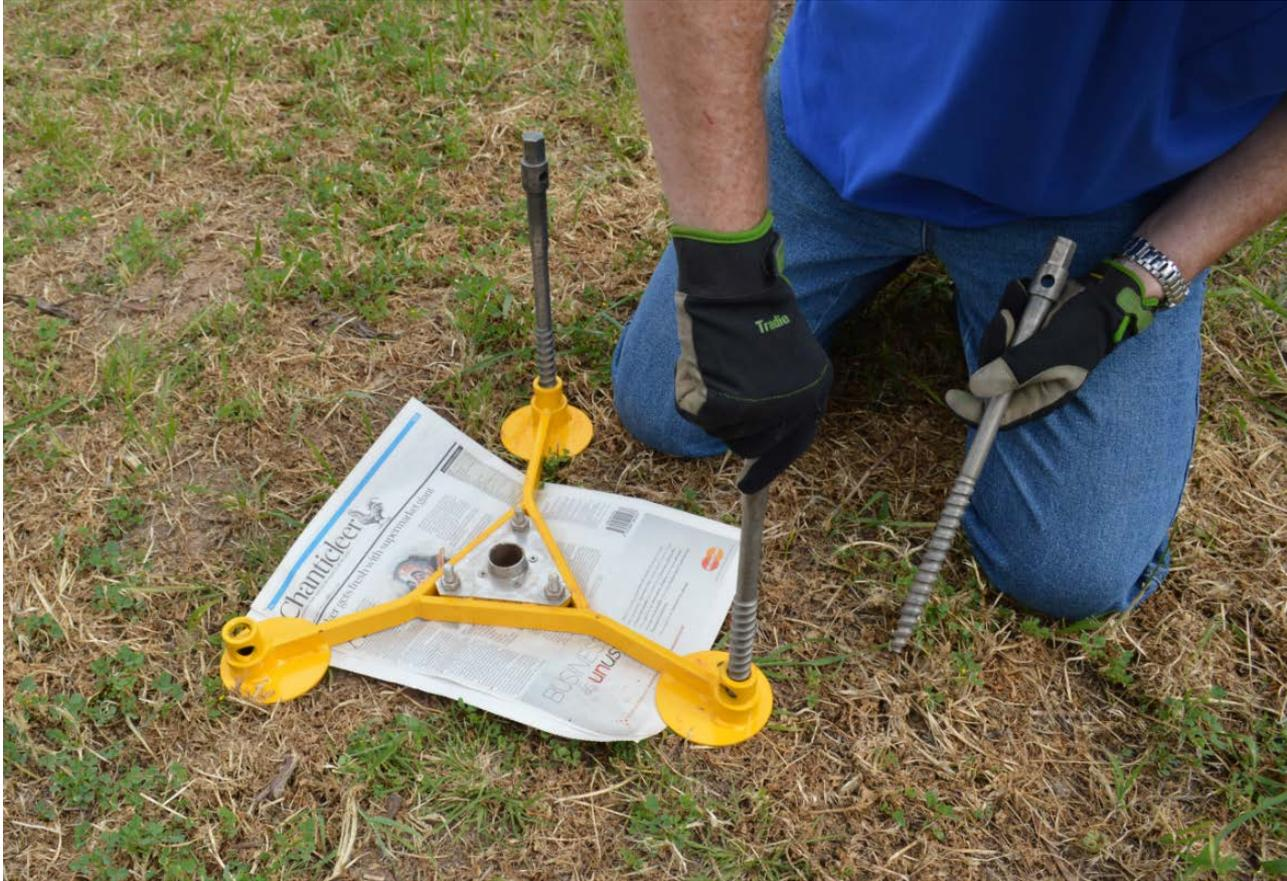
Insert the Screw Pins.
